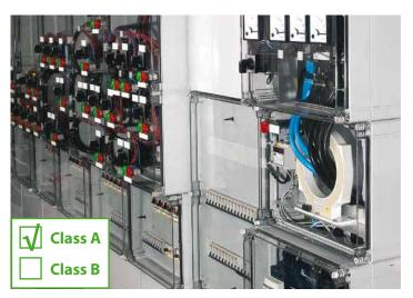
Only Class A terminals are suitable for feed-in lines.
