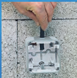
2/ Insert the cable through the end cap
