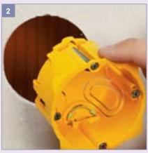
Retractable fixing claws for a better comfort during installation
